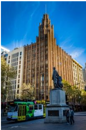
Manchester Unity Building, Melbourne
