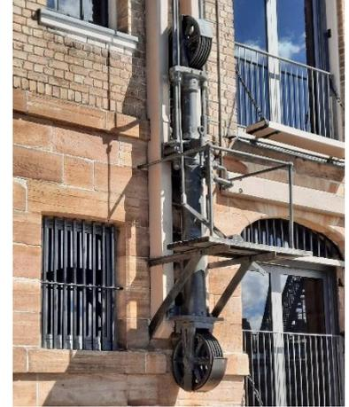
Campbell Storehouses housed imports such as sugar, tea, and spirits from India. Pulleys that were used to hoist cargo can still be seen on the upper levels of the warehouses.
