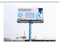
The billboard works through a reverse osmosis system, capturing the air humidity, condensing and purifying the water. After purification, the water flows down into a 20-litre storage tank at the base of the billboard. Water is dispensed by tap. The billboard only costs about \$1200 to install.
