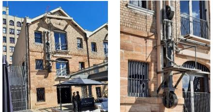
Campbell Storehouses housed imports such as sugar, tea, and spirits from India. Pulleys that were used to hoist cargo can still be seen on the upper levels of the warehouses.
